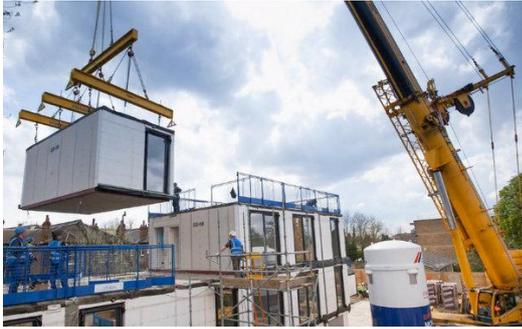
**Fig 1: Installation of Modular Housing**
